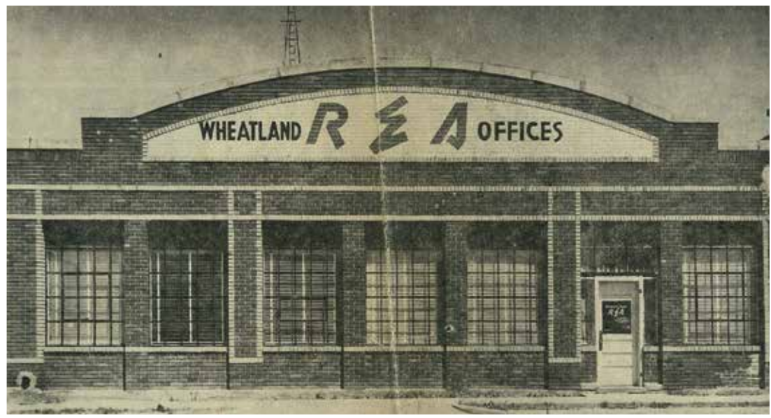
REA Headquarters on August 14, 1952: 893 Members and 655 Miles of Power Lines.
